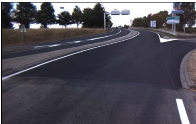
Figure 5: Darker pavement improves nighttime visibility distance under headlight illumination.
