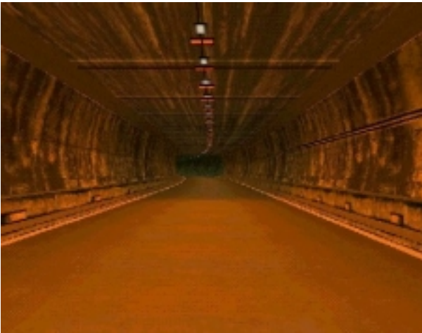
Fig. 5 : The Fourvières tunnel: entrance section
